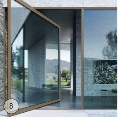
8 LOW IRON GLASS WITH BROWN ALUMINUM FRAME
